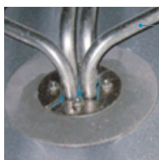
The Roxtec R frame penetration seal can handle several pipes through the same opening.
