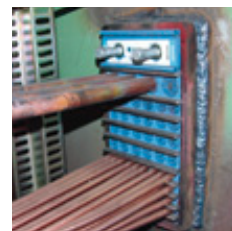
Roxtec S frame transits for multiple pipes in bulkheads or decks.
